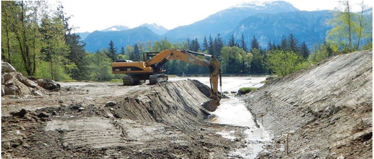
Construction preparing for the new box culverts. (Credit: Squamish River Watershed Society)
