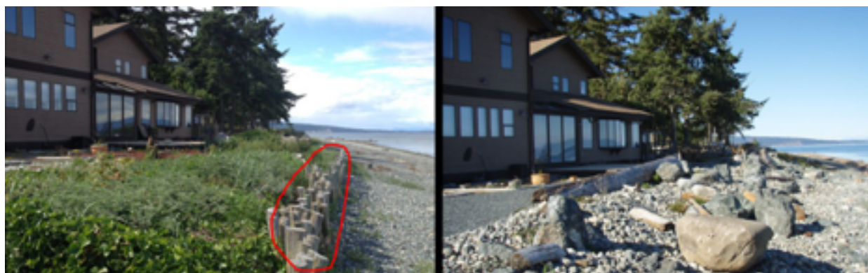
A Green Shores project on an eroding shoreline in Qualicum Bay, Vancouver Island. Left – before restoration. The red line encircles a failing wooden bulkhead where erosion was beginning to undermine the structure. Plants were non-native species. Right – after restoration. The wooden bulkhead was removed, and the shore was regraded to a more natural slope. Large boulders were placed at ~1 m depth and infilled with smaller rock, sand and gravel, to provide a growing medium for native plants. Logs were buried along the upper portion of the shore to mimic the natural shoreline and provide shelter for plants to grow (Photo credit: Green Shores).
